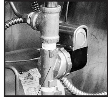
Typical cooling solenoid valve on RK units
